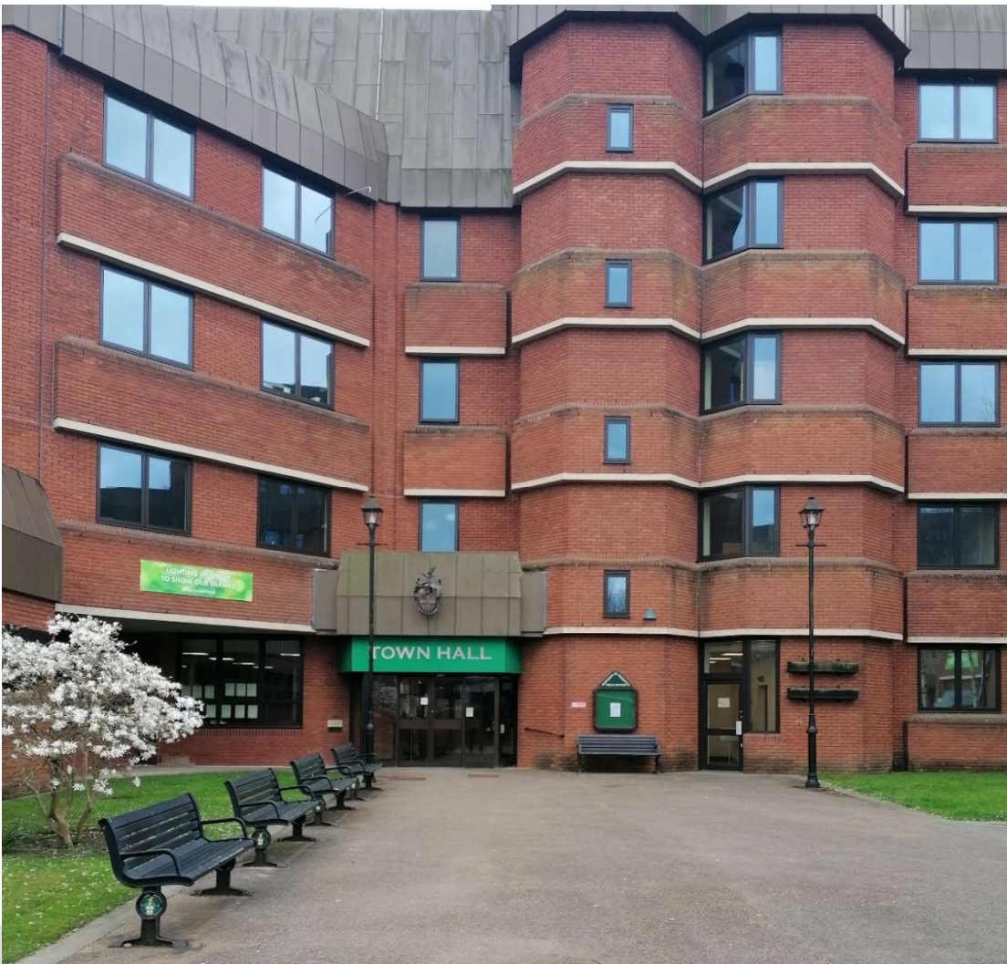
Figure 5: Redditch Town Hall
